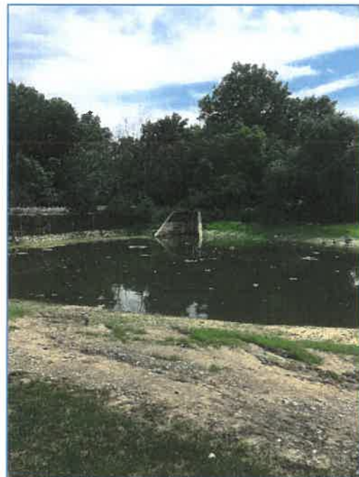
Photo 2: Pond outlet structure, looking SW from easterly side of pond
