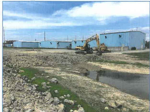
Photo 4: Filled pond, looking NE from westerly side of original pond
