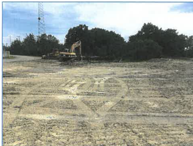
Photo 3: Filled pond, looking S from northerly end of original pond
